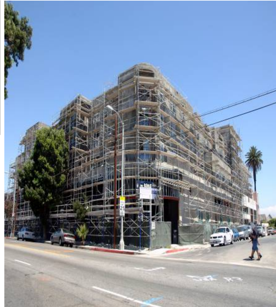
Central Village Apartments (84 units)
